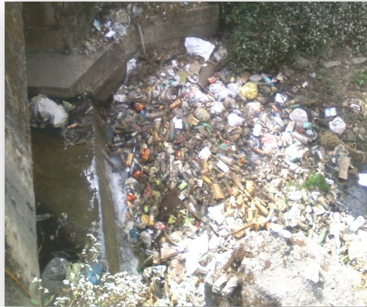
Low lying drains clogged with solid waste, now used as dumping space
